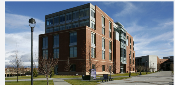
WASHINGTON STATE UNIVERSITY - PHASE 1 DATA CENTER
